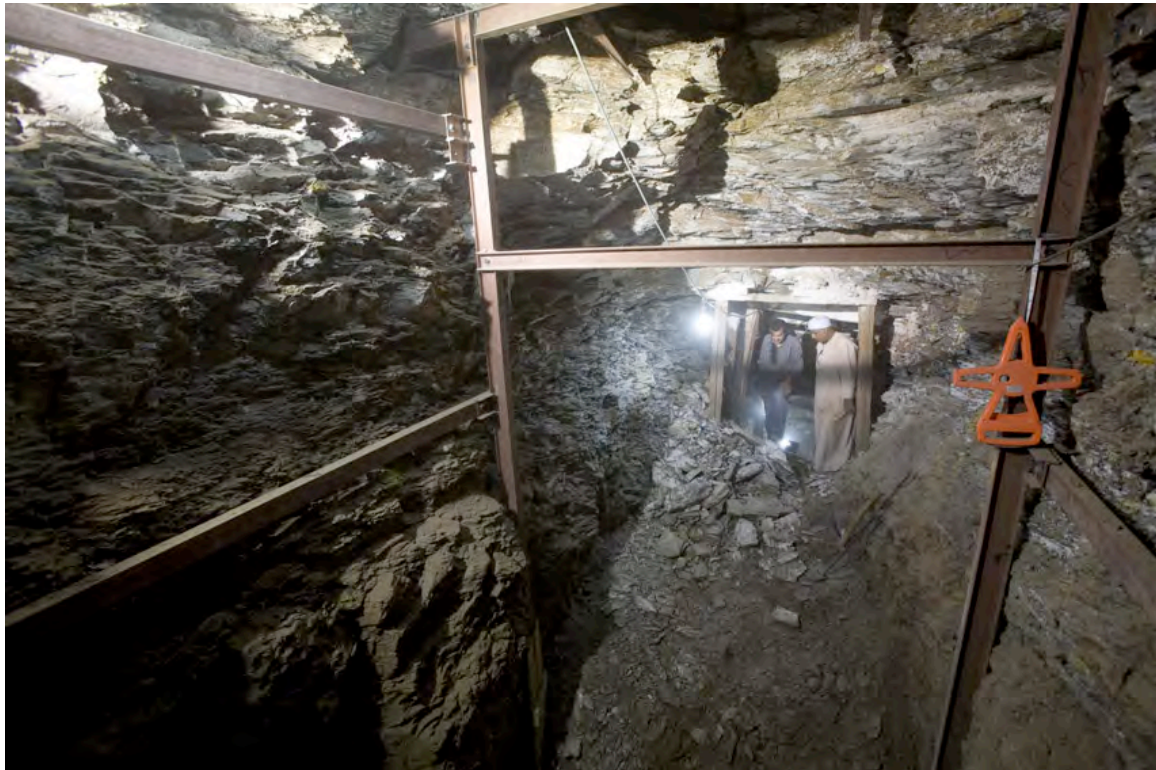
A steel reinforcement structure supporting the ceiling of the tunnel.
